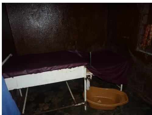
Figure 53: Bo district CHP delivery room
